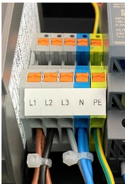
Connection is done via the terminals L1, L2, L3, N and PE of the terminal block.
