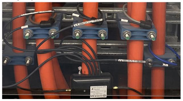
The connection housing of a current module can be fixed directly to a cable using cable ties.
