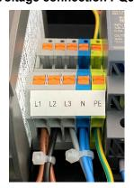
Connection is done via the terminals L1, L2, L3, N and PE of the terminal block.
