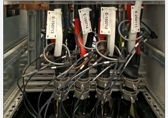
Field installation of Current Link modules
