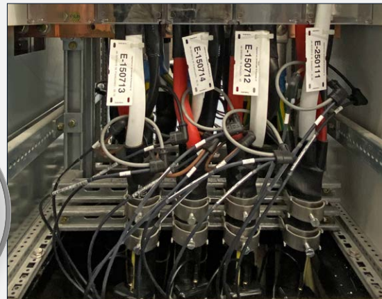
Representation of the Current Link modules for individual power curve measurement/channel
