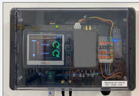
Detailed view of the decentralized mounted base stations LINAX® PQ5000CL
