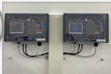
Representation of the Current Link modules for individual power curve measurement/channel
