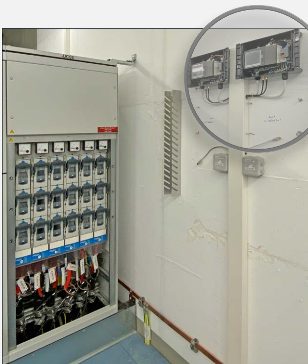
Representation of the switchgear and the decentrally mounted LINAX® PQ5000CL base stations
