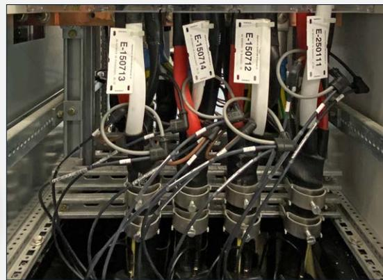
Installed Current Link modules per feeder
