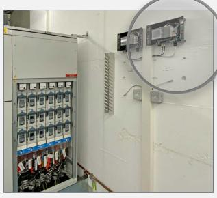
Representation of the switchgear and the decentrally mounted LINAX<sup>®</sup> PQ5000CL base stations
