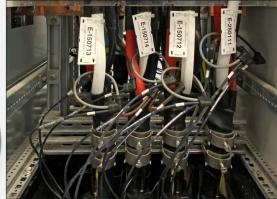
Installed Current Link modules per feeder
