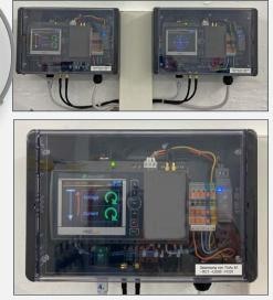
Detailed view of the decentralized mounted base stations LINAX® PQ5000CL
