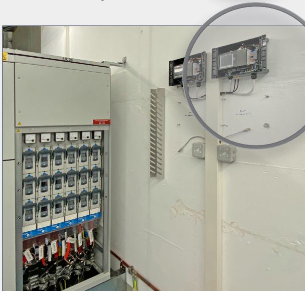
Representation of the switchgear and the decentrally mounted LINAX® PQ5000CL base stations
