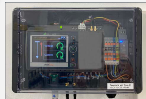
Detailed view of the decentralized mounted base stations LINAX® PQ5000CL
